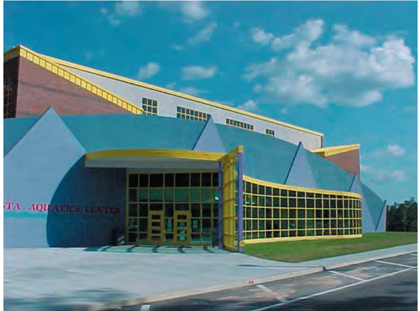
Aquatic Center in Augusta, Georgia
